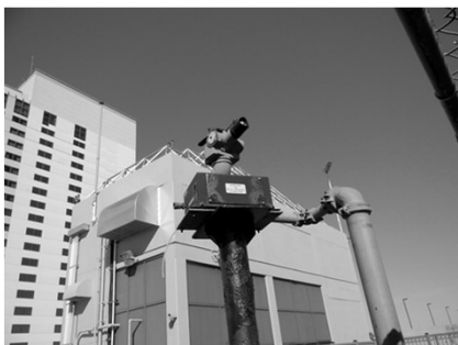
FIGURE 14.16 Firefighting automatic remote monitor nozzle with 10-minute foam concentrate supply. Courtesy of J. M. Foley
